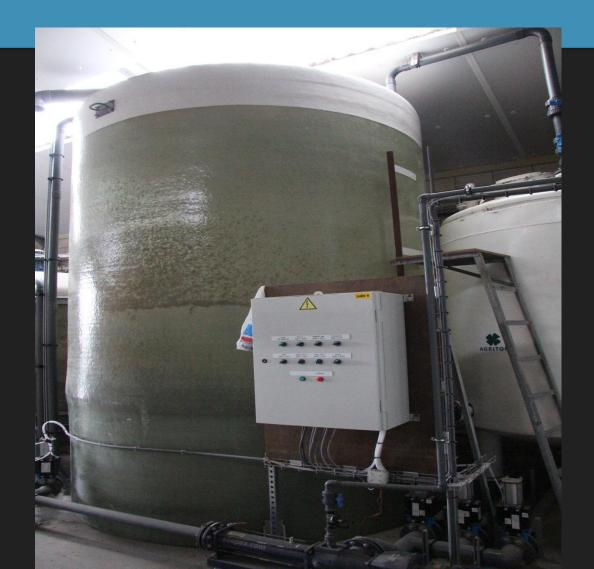
Storage tank after min: 24h of fermentation Check point PH=3
