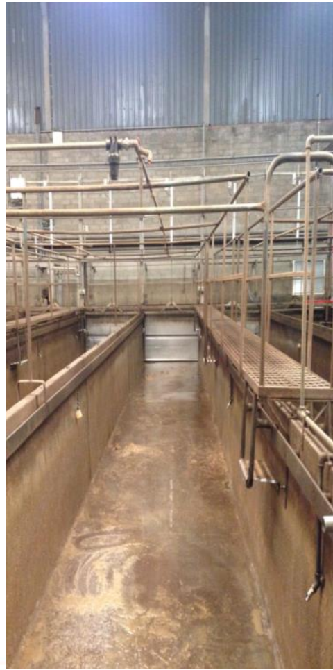
Before Power Wash
