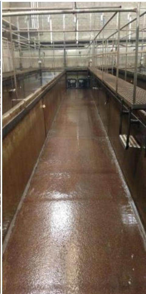
After Power Wash
